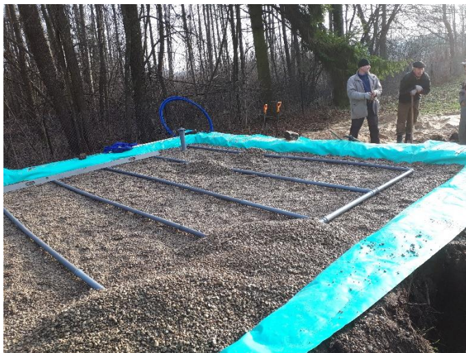
Figure 12. Infiltrating drainage in the backfill
